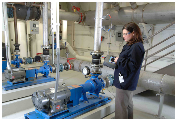
Figure 4: Clamp-on ultrasonic flow meters can be used for troubleshooting a wide range of flow issues, from verifying the reading of another meter to monitoring flow systems over an extended time period.
