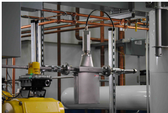
Figure 3: Coriolis flow meters are designed to directly measure fluid mass over a wide range of temperatures with a very high degree of accuracy.
